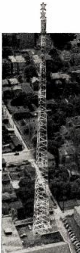
WAVE-TV, Louisville, Kentucky. Truscon Self-Supporting Tower, 569 feet high.
