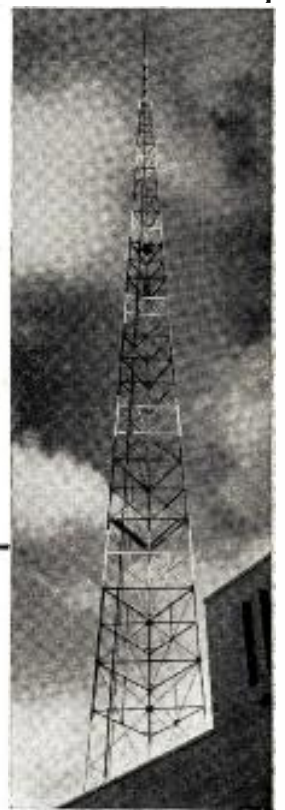
WOW, Omaha, Nebr., Truscon Self-Supporting AM-FM-TV Tower, 500 feet high overall.
