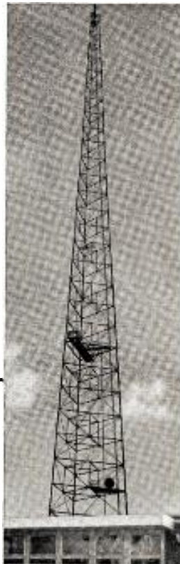
WXEL-TV, Cleveland, Ohio. Truscon Self-Supporting Tower, 437 feet high.
